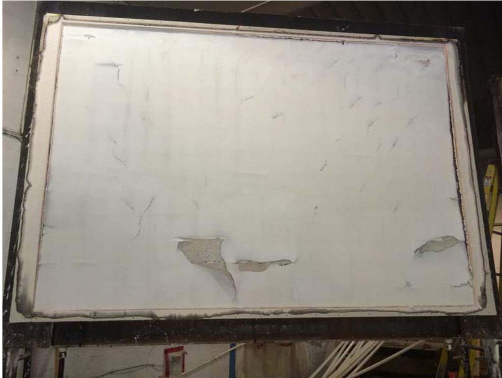
Figure 9: Exposed side at termination of fire exposure.
