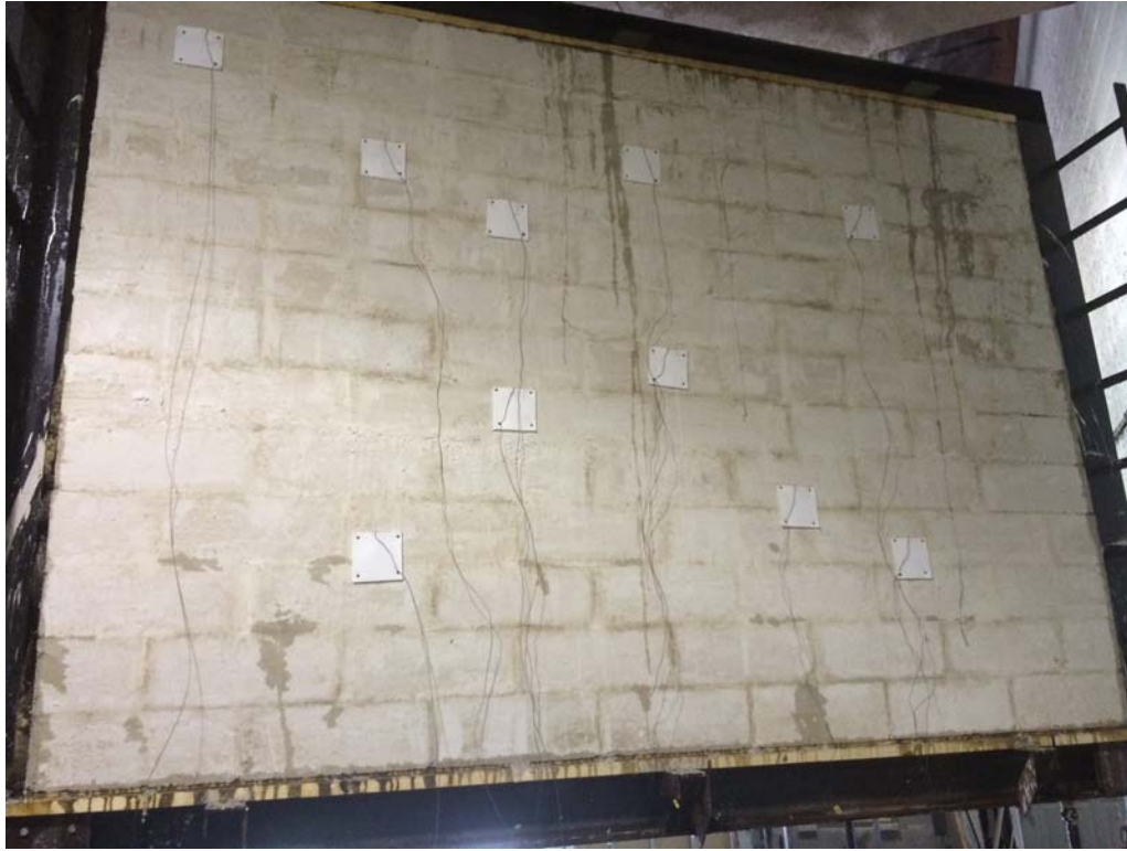
Figure 11: Unexposed side after the hose stream test.
